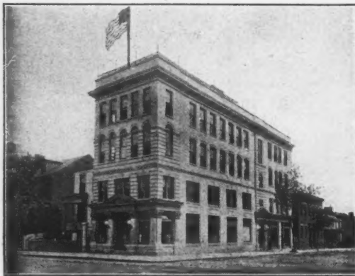
Future Home Office Southern Aid Society of Va., Inc. N.W. Cor. 3rd & Clay Sts. Richmond, Va.
